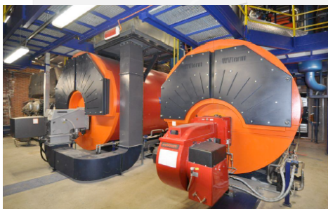
New gas hot water boiler rated at 7 MW and 10 MW
